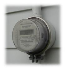
This question has plagued home inspectors and Realtors for a while now. I hope to help answer this question. The problem comes when a 60 amp meter socket is in place and someone has upgraded the panel to 100 amp service. The round meter socket may be an indication of an electrical upgrade without permits. Typically if there is an upgrade
