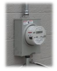
meter socket is 60 amp and the grey meter socket is actually a 100 amp round meter socket. Grey socket measures 2-3/4" and the red one measures 2".
