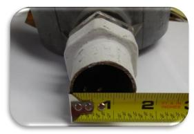
Electrical code dictates what size wire (and how many) you can run in a raceway. This is all based on heat as we don't want too many wires jammed in to one pipe and they are all hot (temperature hot not electrical hot). Some air is required to cool the wires thus the reason the raceway is oversized to the wires contained.
